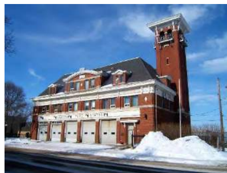
Figure 22: Fire Hall before renovations
