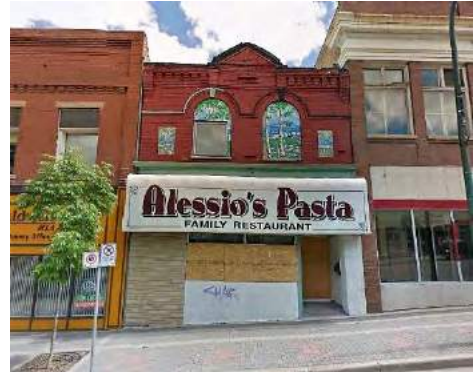
Figure 24: 121 10 th Street before renovations
