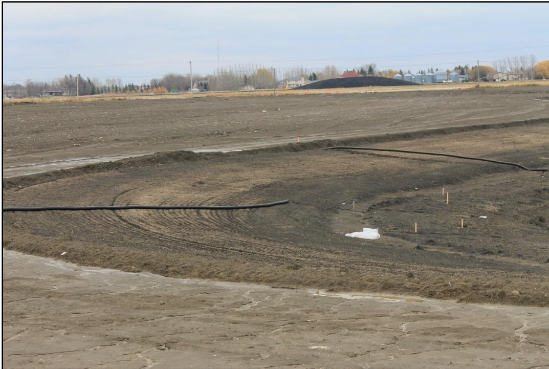
Figure 6.1. Earth dyke installed to redirect surface runoff towards an NSP.
