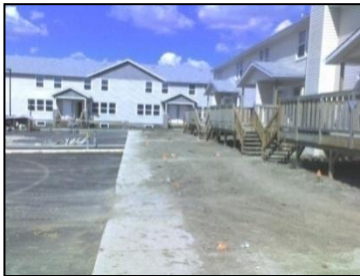
Re-used McNab Park Housing sold through the Mortgage Flexibilities Support Program, 209 Camponi Place
