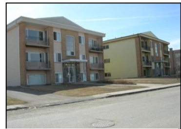
Cress Housing's Hopkins 2 Project, 604 Hopkins Street
